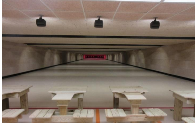
Firing Range at Auburn CF Project Cost: $9.5M
