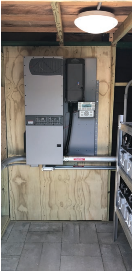
▲ DEC installed an 8 kW off-grid solar system at the Narrow Island Campground caretaker's cabin in Lake George. This project powers the facility with clean renewable energy and improves power resiliency.
