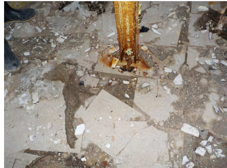
Photo 229: Building 1 Basement - Typical base of rotunda floor shoring
