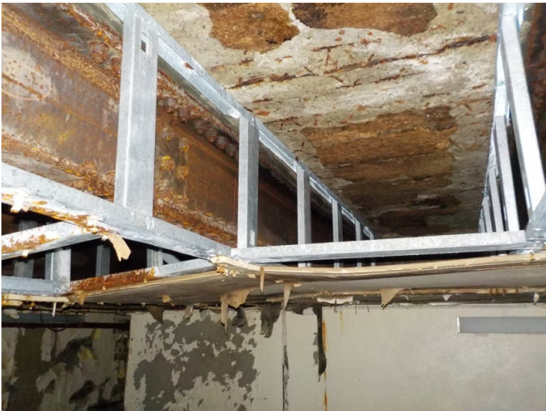
Photo 235: Building 1 Basement - Framing under kitchen coolers
