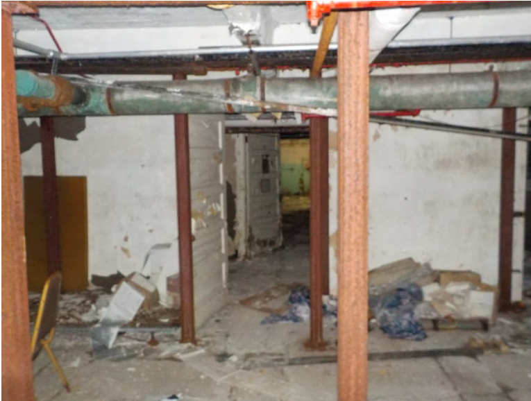
Photo 222: Building 1 Basement - Typical west side shoring of rotunda floor
