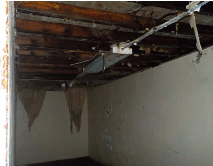
Photo 231: Building 1 Basement - Floor framing at kitchen storage
