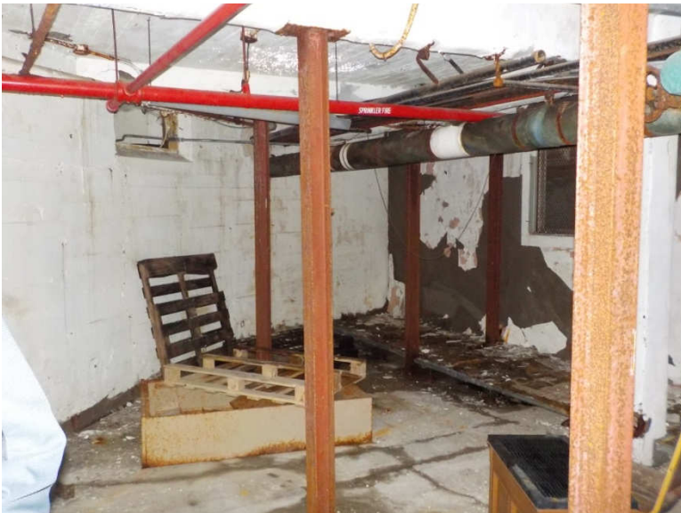
Photo 223: Building 1 Basement - Typical west side shoring of rotunda floor
