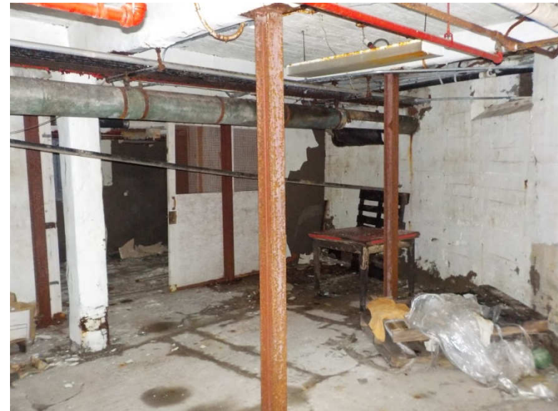
Photo 221: Building 1 Basement - Typical west side shoring of rotunda floor
