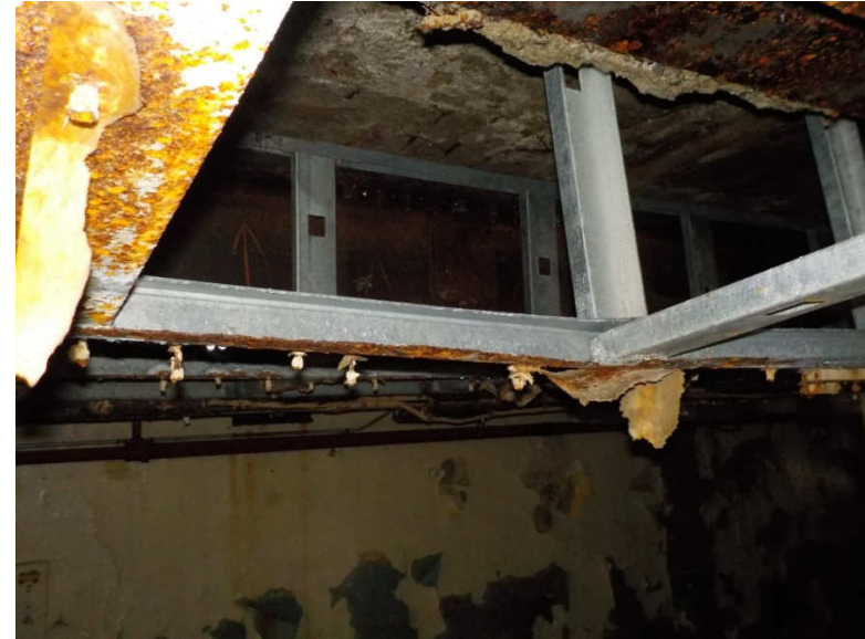
Photo 236: Building 1 Basement - Framing under kitchen coolers
