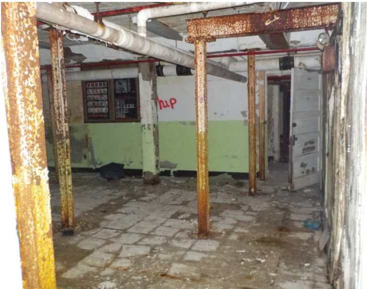
Photo 227: Building 1 Basement - Typical east side shoring of rotunda floor
