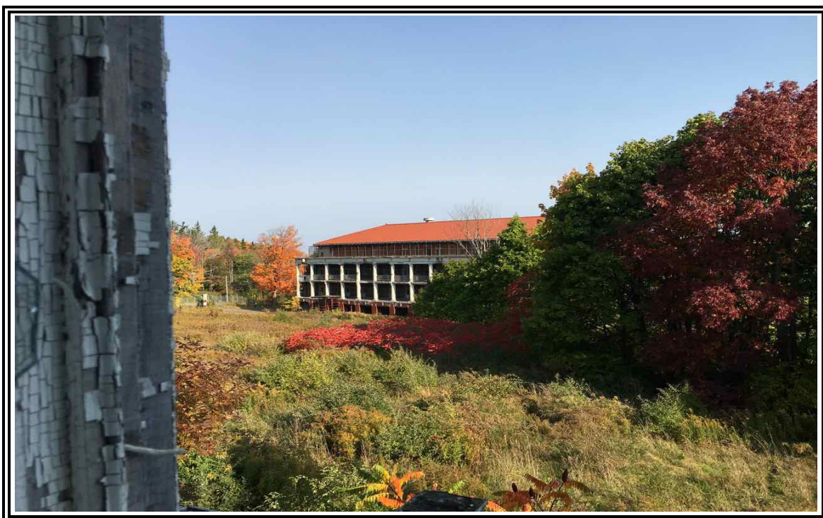
Exterior of Typical Buildings Peeling Paint – Likely Lead-Based
